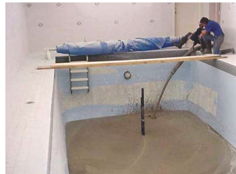
Prairie's FlowFill is best suited to areas that safety or physical constraints hamper compaction.
