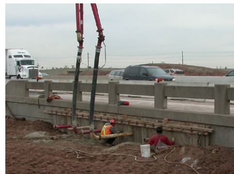
Prairie's FlowFill is best suited to areas that safety or physical constraints hamper compaction.
